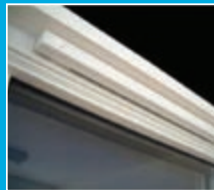
Improve air flow by leaving trickle vents open on all windows or leave windows open (if safe)
